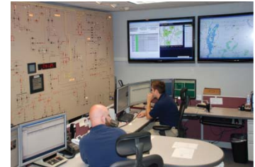
Vermont Electric Cooperative's Smart Grid Operations Center
