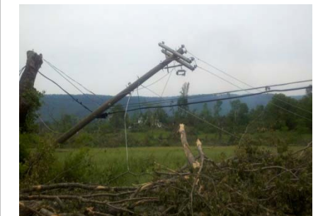
April 2011 Storm Damage
